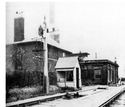
Engine house at the top of the Swannington Incline (now demolished)
