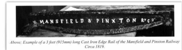
Above: Example of a 3 feet (915mm) long Cast Iron Edge Rail of the Mansfield and Pinxton Railway Circa 1819.
